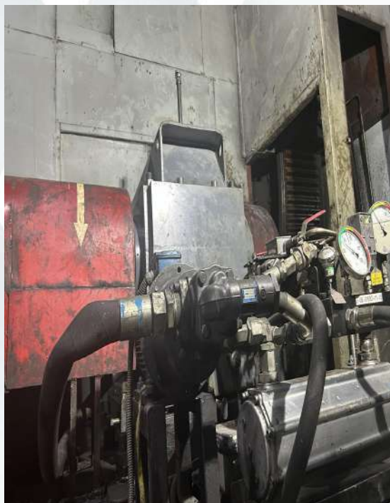
Huadian International Fengjie Power Plant
